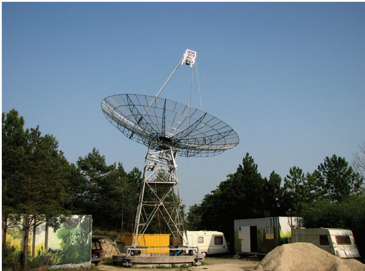
*Parabolic antenna built by the author. Diameter = 10.50 m*
